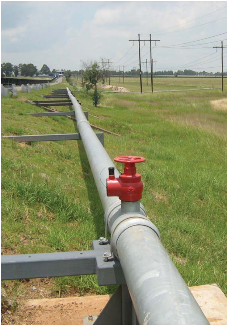
Installed Lula™ Pipeline
