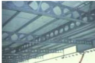
Simply supported tapered beams in a pitched roof minimize building height.
