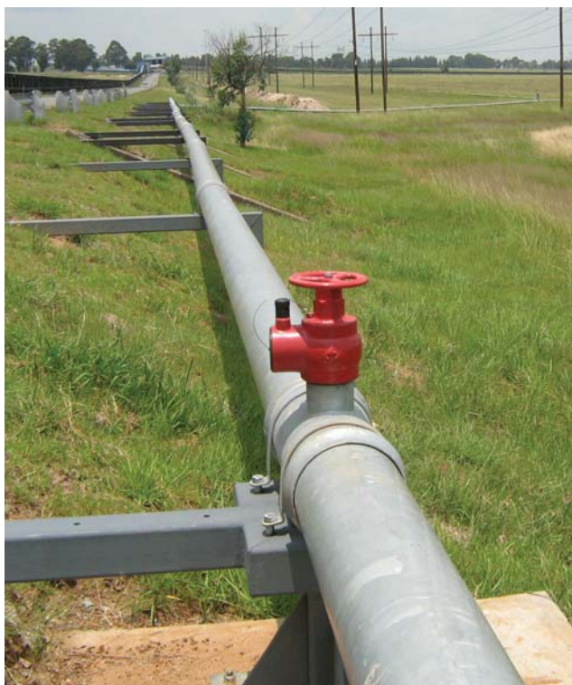
PVC pipe fits into Lula™ steel pipe - various lengths available
